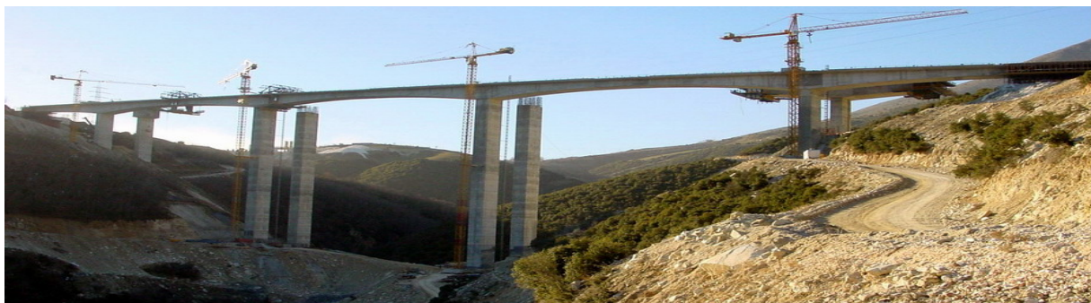
Figure-8: G12 bridge during construction
