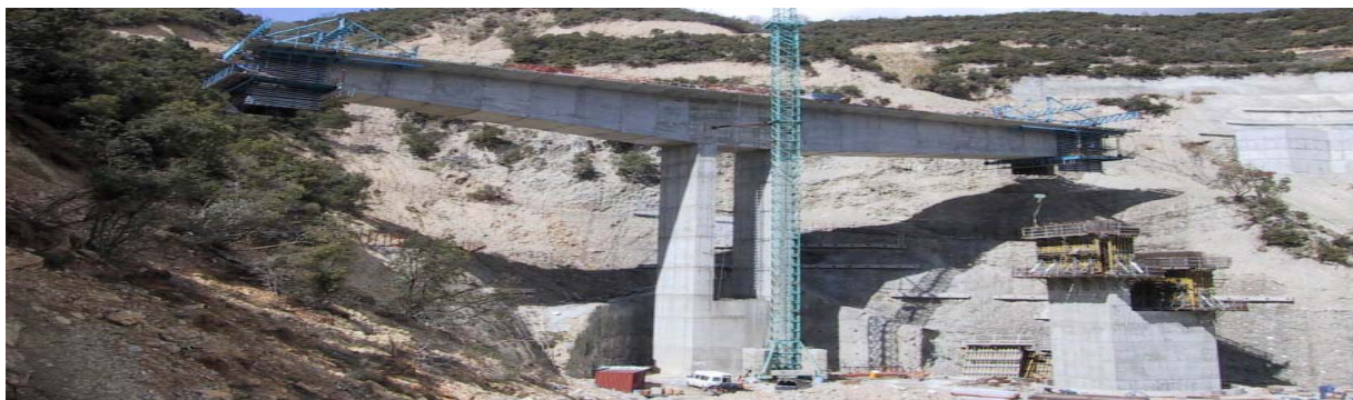
Figure-3: G2 bridge during construction
