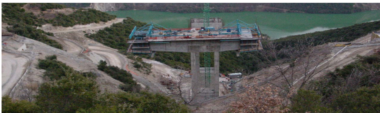
Figure-2: G1 bridge during construction
