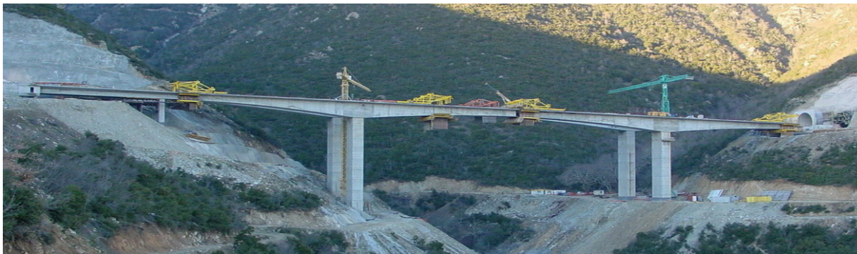
Figure-6: G10 bridge during construction
