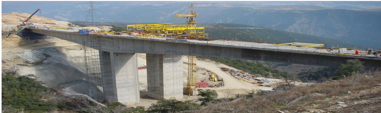
Figure-4: G9 bridge during construction
