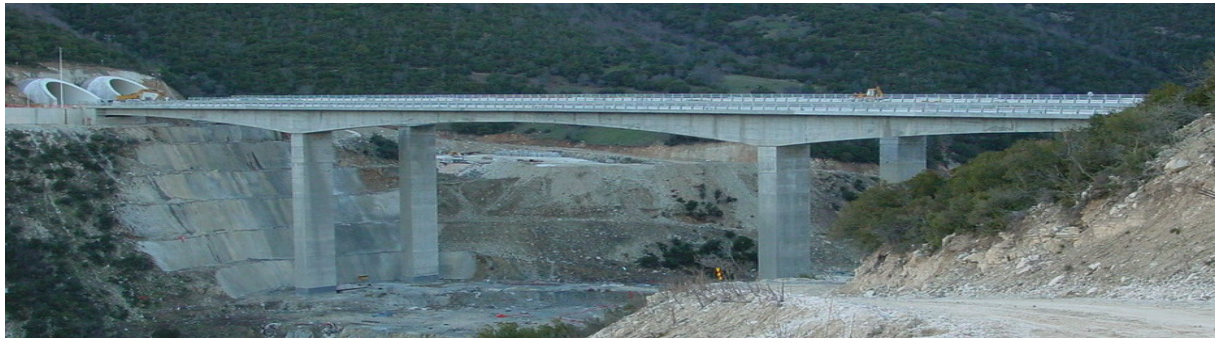
Figure-7: G11 bridge during construction
